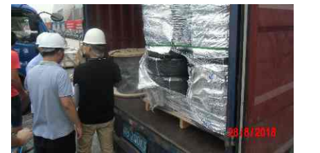
(弱电电缆进场前验收)
